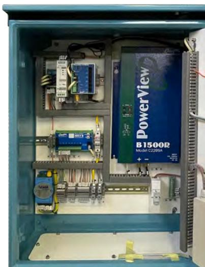
An example of a single output 30V/50A switch mode T/R in wall mount enclosure
