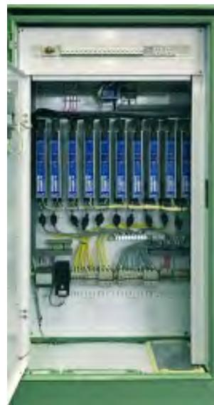
Example of a 15V/400A T/R consisting of 10 individually controllable anode outputs of 40A each.
