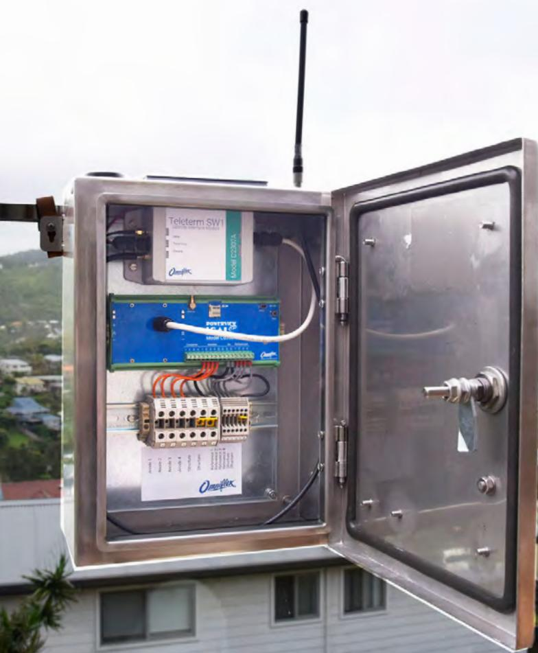
A recent case study of the iGAL/SW1 combination has been its deployment for the monitoring of a galvanic cathodic protection installation of a steel culvert under a highway in Far North Queensland, Australia. In this application, the system allowed asset managers to monitor the protection of the steel culvert without the need to physically visit the remote site to conduct costly and time-consuming CP testing, which could all be done remotely.
