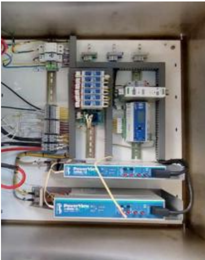
Interval view of TRU's and controller
