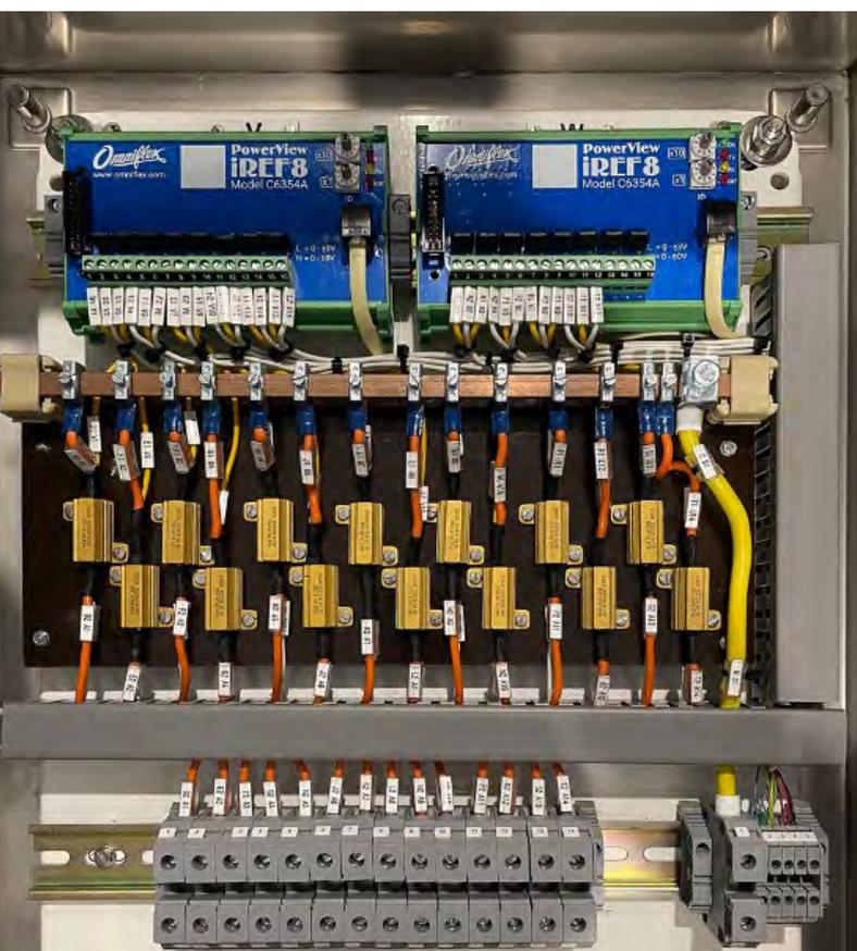
DC with an accuracy of 0.2 per cent and an input impedance of greater than 100 Mohm. This versatile module can also monitor current shunts as low as 50 mV and T/R voltages as high as 60 V making this an ideal module for monitoring existing CP systems with minimal intervention. Each input has surge protection to protect the inputs to surges in excess of 60 V.
