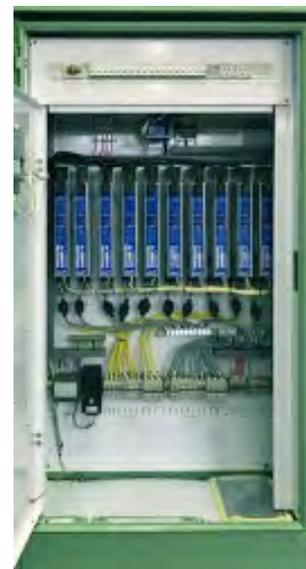
Example of a 15V/400A T/R consisting of 10 individually controllable anode outputs of 40A each.
