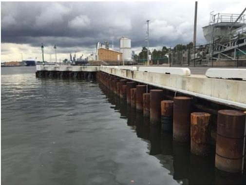
*A typical sheet steel pile wharf with distributed PowerView CP system installed*
