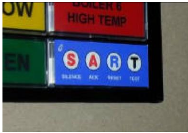
Location of SART fitted to Annunciator
