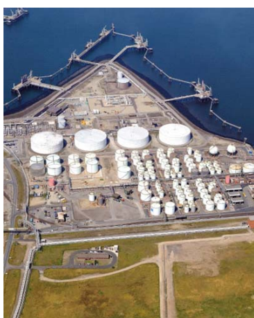
Seal Sands Tank Farm protected by Omniflex alarm systems.
