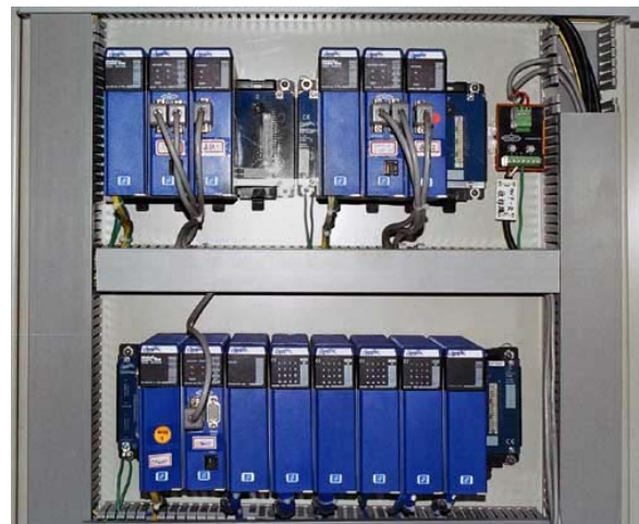
A MAXIFLEX dual redundant CPU system
